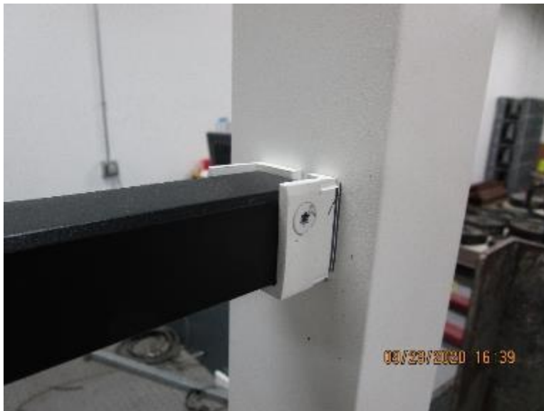
Photo No. 8 Cast Aluminum Rail Bracket
